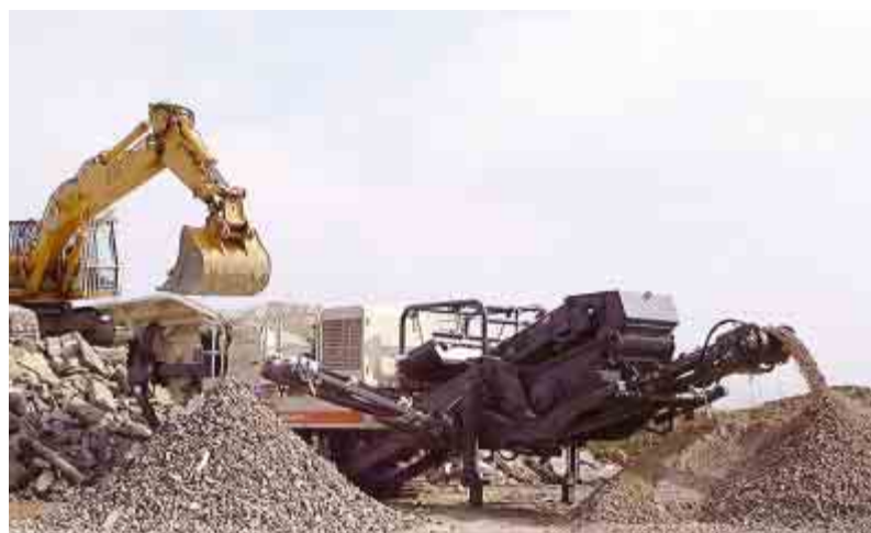
The Lokotrack crushing recycled concrete in Germany.
